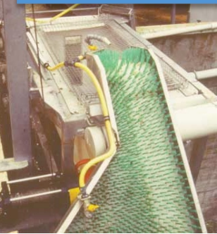
Upstream passage facilities
