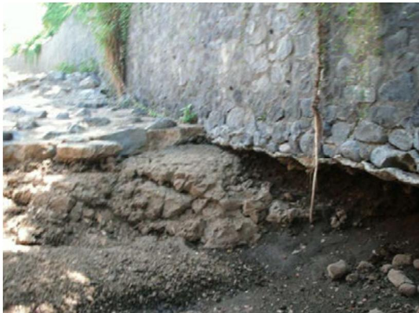
*Photo n°30 – AFFOUILLEMENT DU MUR D'ENDIGUEMENT RIVE GAUCHE ET INCISION DE SEUIL AU DROIT DE LA MAISON DE RETRAITE - PK 0,650*
