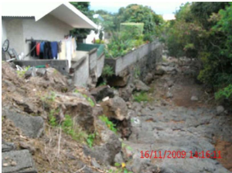
*Photo n°32 – VUE DEPUIS L'AMONT DU MUR RIVE GAUCHE AFFOUILLE AU PK 1,7*
