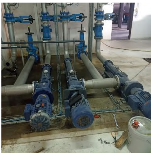
Revamping station de pompage - STEP Runeo
