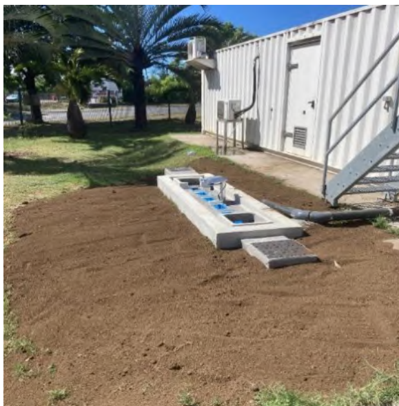
Installation Canal Venturi – Boulangerie Young
